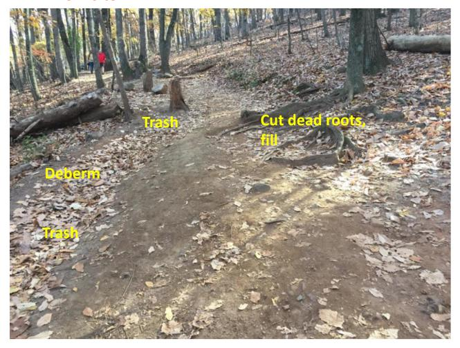
Trash left of little stump. Cut roots and move any rocks that are trip hazards to make trail more attractive. Deberm and trash creep area using material as fill near tree. Also, fill is available from creep areas above.
