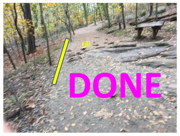
Deberm and place big log (or logs) where creep is occurring and wedge in place. Use deberm material to backfill behind rocks near bench and compact as well as you can using the tamper. Remove trip roots near bench. More fill material is available from worksites above and below.
