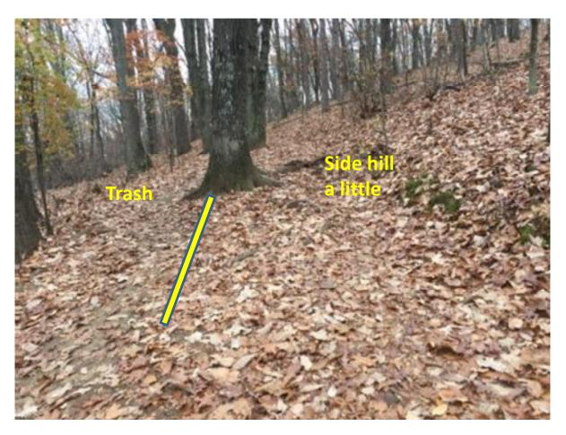
Tread is to the right of the tree. Build a short crib wall and backfill but allow for water to sheet off. Side hill a little near tree. Cut trip root. Backfill around big root near tree. If you can find a good rock or two, bury rock partway in front of root to make a rock dam and backfill behind it so the step over the root isn't so high. Take dirt that has sloughed off to the left and use for fill. Trash left of tree.
