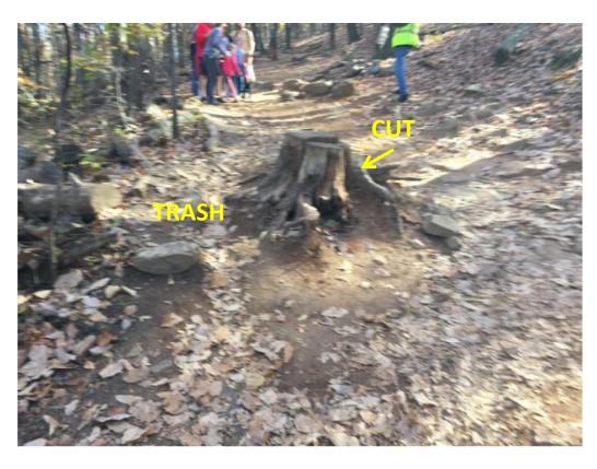
Trash left of big stump above and below —use stump as part of the trash. Cut roots sticking out to the right of stump and move loose rocks to make trail there wider and more attractive. Deberm by moving old log just above stump.
