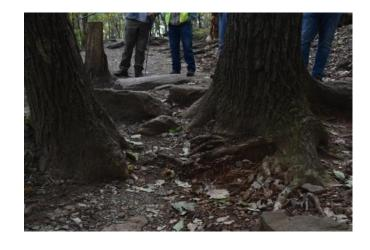
Remove odd rocks, add small step and/or rock dam and backfill to allow hikers to walk single file through he two trees. Use a well graded soil removed above and add organic soil to make tread to resist erosion.
