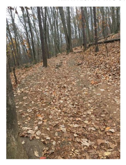
Work at site 15 just above should divert the water that made the rut here. Clean out rut. Dig in rocks into the rut every 8 to 10 feet to make rock dams, backfill, and compact. Trash left of tree. Deberm near tree and build up trail and slope 3 to 5 degrees to the right. Get some fill from the work group up the trail.
